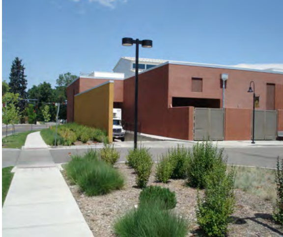
This storage and loading area is located away from the street and is screened from view.
