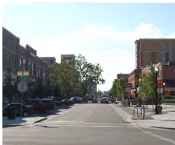
Extended corners protect pedestrians from vehicular traffic by narrowing the street and causing cars to slow down.
