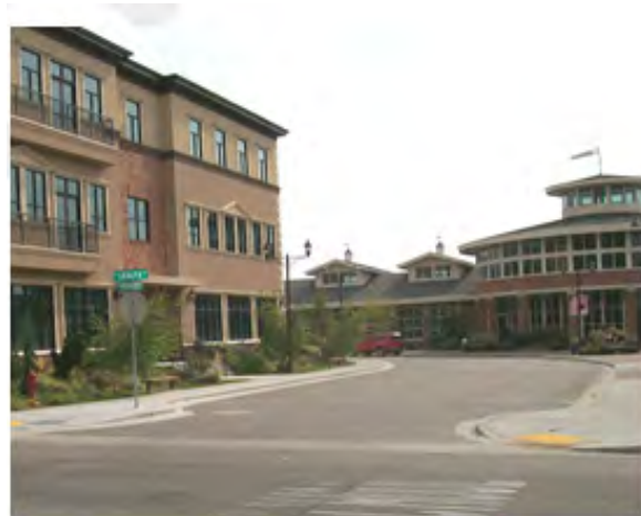
Retail and multi-family residential uses in this activity center are horizontally mixed and well integrated—both visually and physically.
