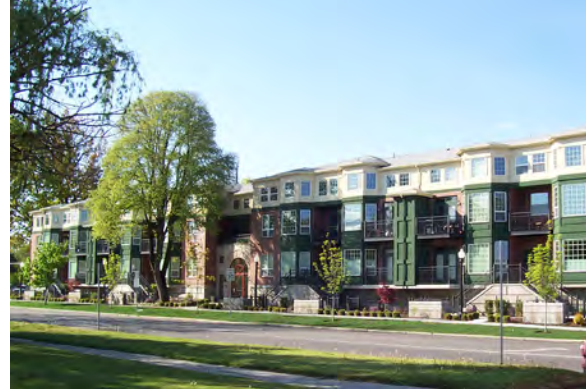
The 30th Street Area Master Plan identifies suitable locations for high density residential development, such as these row homes
