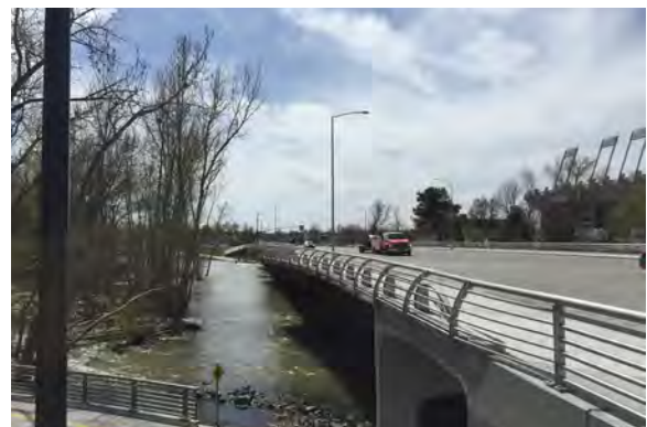
The 2016 Broadway Bridge
