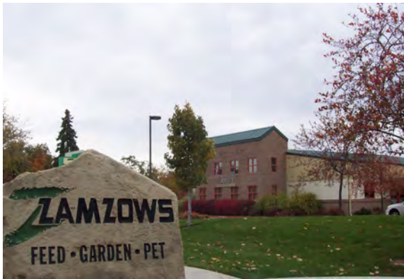
Redevelopment along the State Street Corridor.
