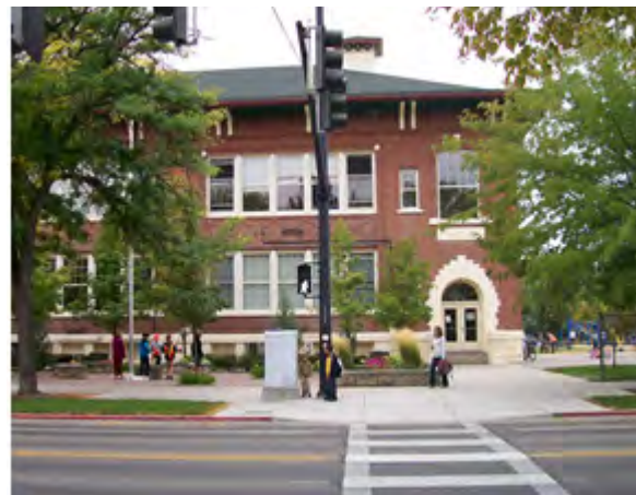
The architecture and landscaping of this school helps to blend it in with the neighborhood.
