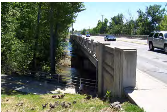
The 1956 Broadway Bridge
