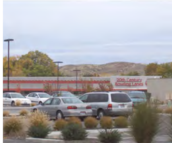
Façade improvements and landscaping can help improve the appearance of existing centers when major rehabilitation is not feasible in the near-term.
