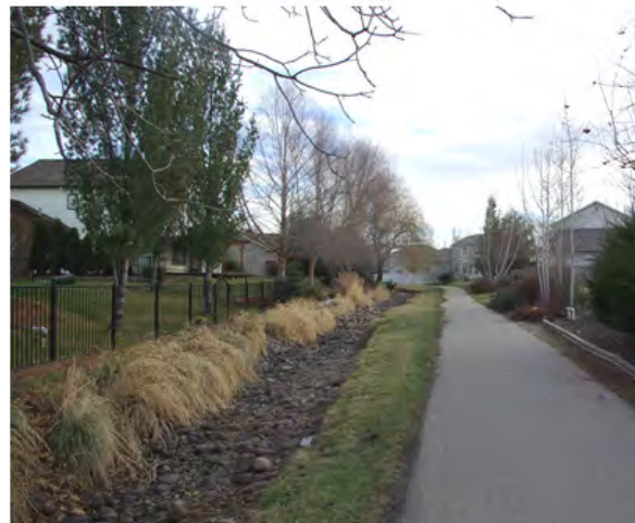
On-site retention helps purify water before it becomes ground water.
