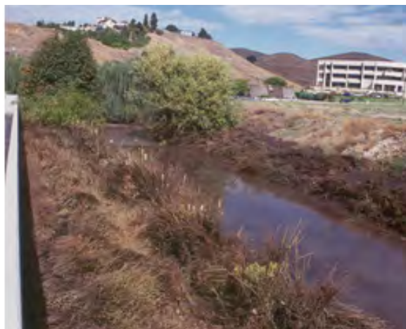
Flood control improvements help reduce runoff during flood events.
