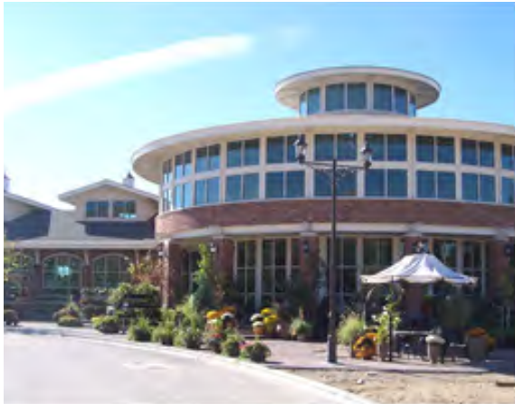
The 36th Street Garden Center received a Silver LEED certification from the U.S. Green Building Council for its sustainable design.
