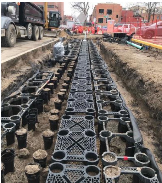
Figure 21: Photographs of Grove Plaza during the installation of a suspended pavement system to support tree growth, and the same plaza five years later.
